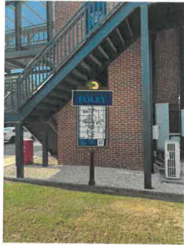
West Pedestrian Bridge pin #24278
