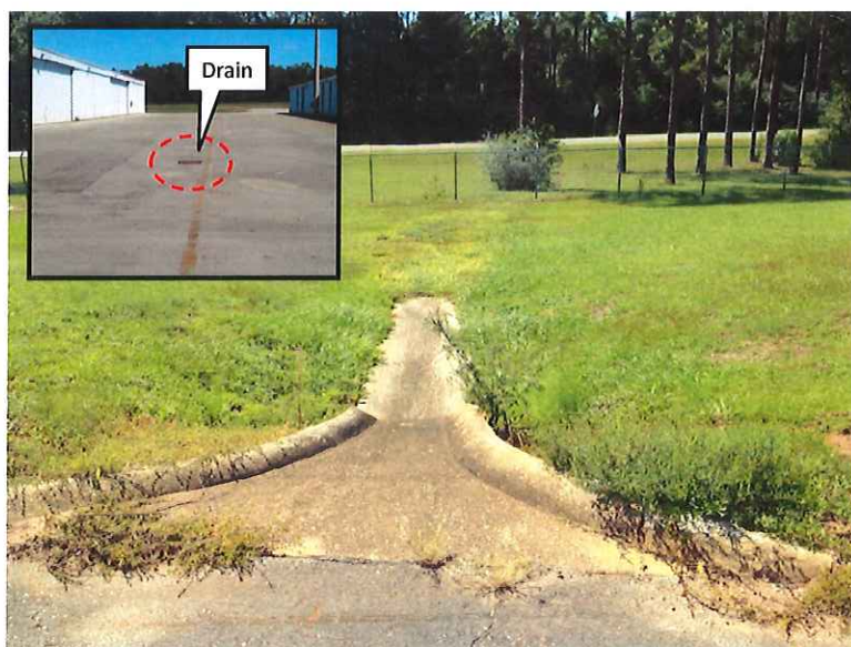
Storage building and parking area drainage along western portion of facility.
