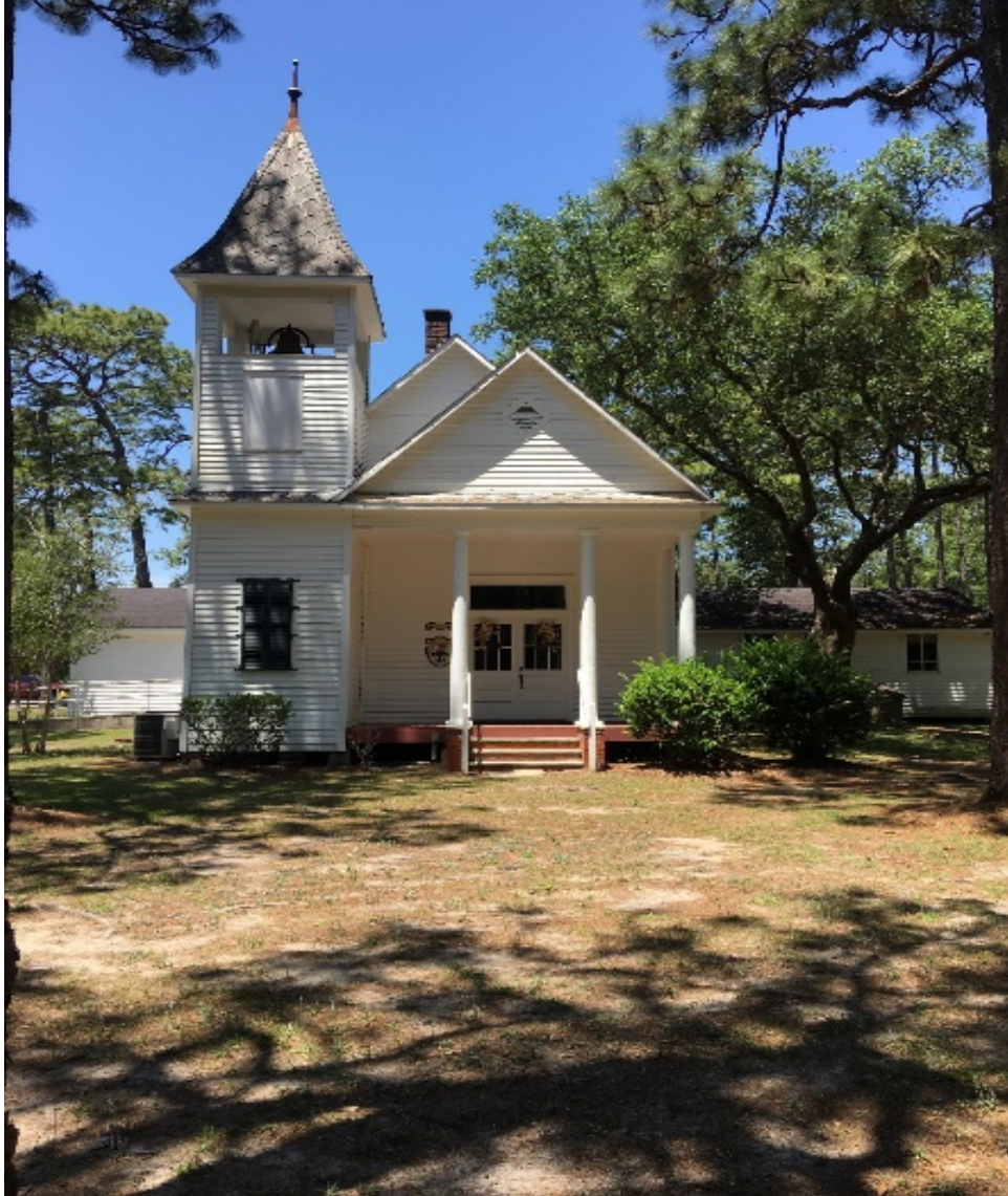
Figure 4.15 Swift Presbyterian Church, Listed on the National Register of Historic Places
