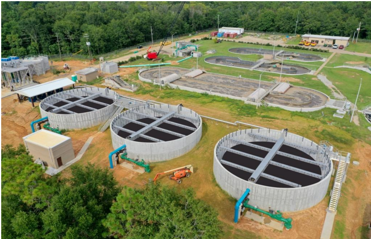
Figure 5.3 Riviera Utilities Wastewater Treatment Facility
