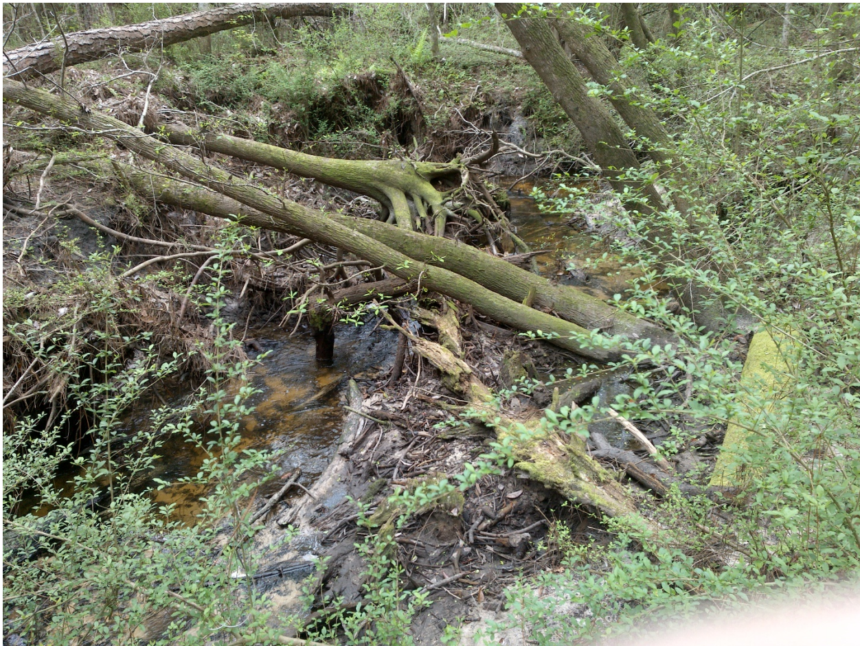
Figure 7.11 Bank Erosion/Sedimentation Within Hammock Creek
