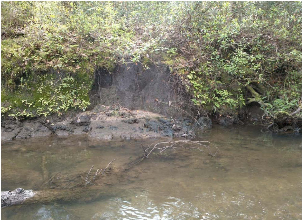
Figure 7.8 Bank Sloughing Along Wolf Creek
