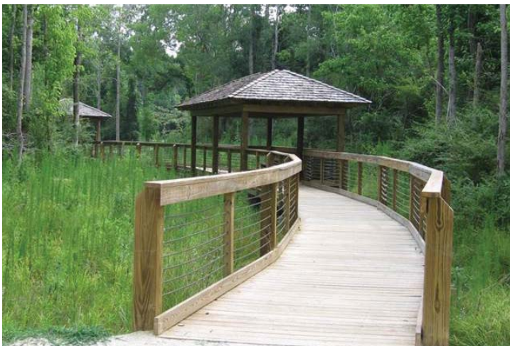
Figure 15 - Character image featuring Town Creek Park in Auburn, AL. This is a great example of how to provide access through a wetland without being overly intrusive to the existing habitat.
