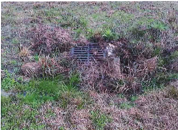
Existing Drainage Structure
