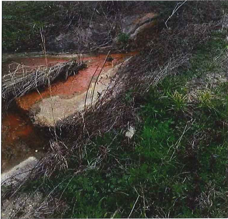
Existing Drainage Structure
