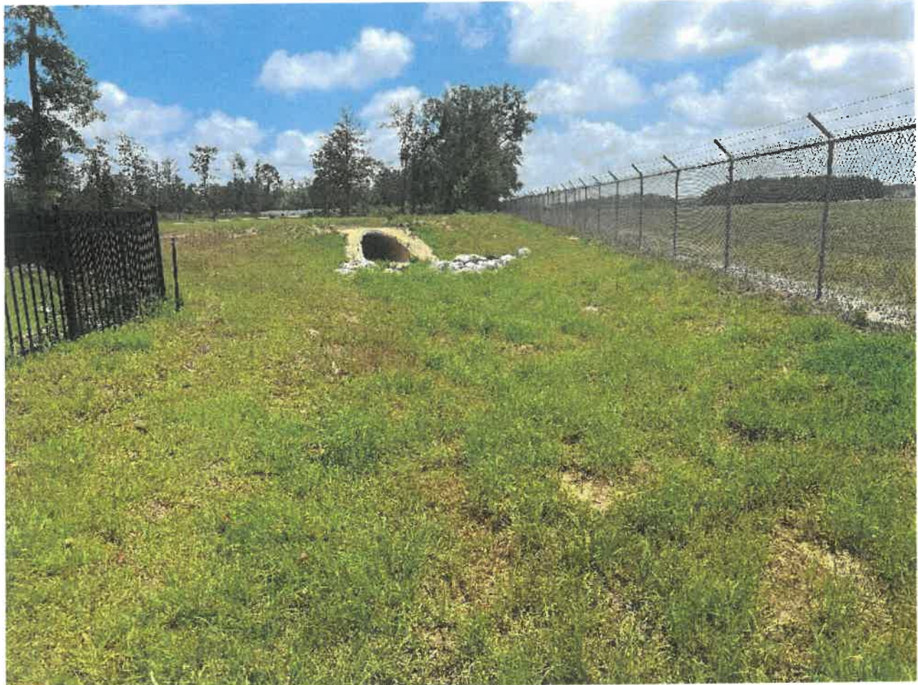
3. Area near outfall does not appear to be overgrown
