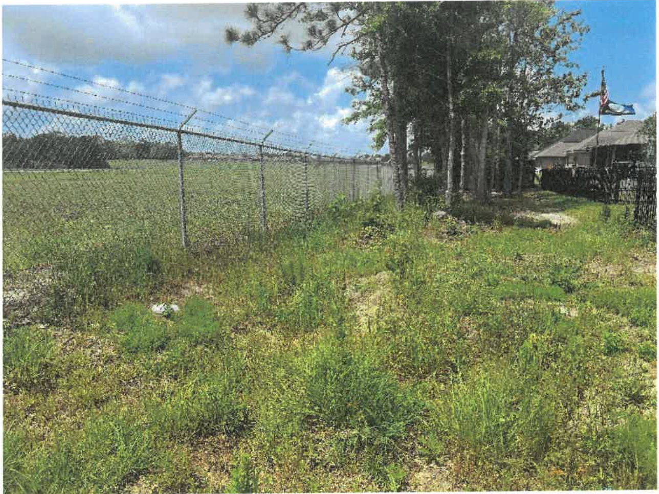
2. Some weeds in common drainage area
